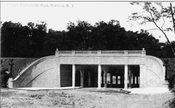
The Parkside Aqueduct carries the canal over Parkside Avenue.
