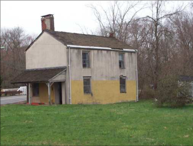
The bridge tender's home before restoration.
