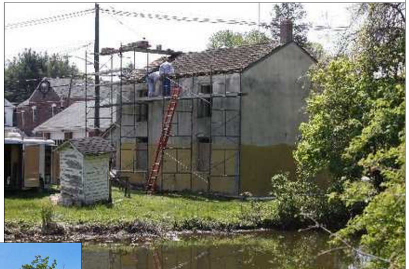
The home during restoration
