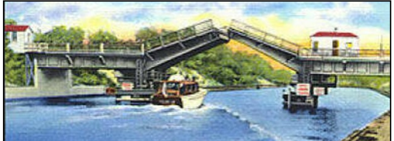
Heading south through the original Rt. 88 bridge on the Point Pleasant Canal.
